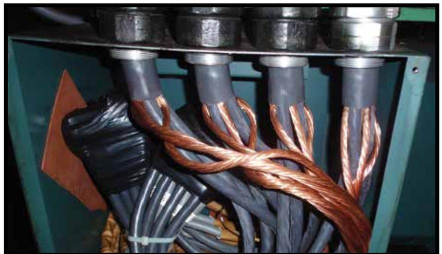
single factor in VFD cable performance is the effective impedance of the ground system (at the frequencies of the generated current noise), selection of cables that optimize the total ground potential copper and conductor surface area (for high-frequency performance) can result in a significant reduction in common mode current and its harmful effects.
